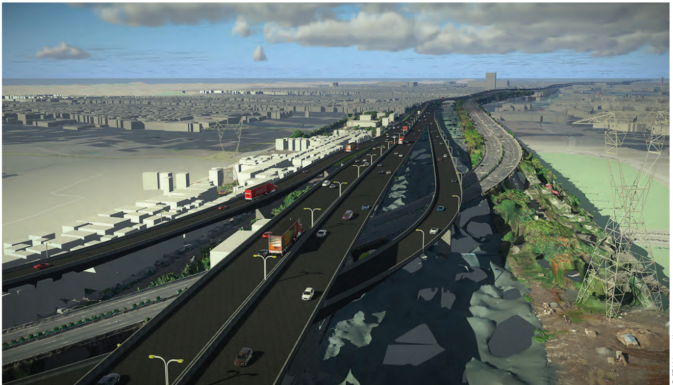
PT Wijaya Karya is performing design review on the project. The double-decker design was chosen to make the best use of a site constrained by heavy traffic, surrounding buildings, road interchanges, railroads, and waterways, as well as underground and intertwined gas pipelines, water pipes, and optical fibre lines.
