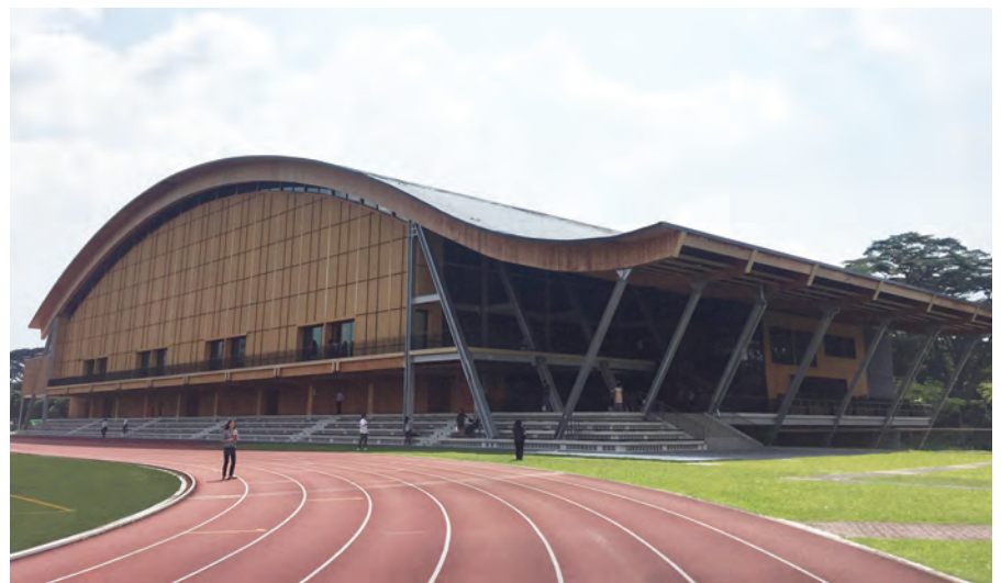
LEFT AND BELOW: The Wave is the sports hall at Singapore's Nanyang Technological University constructed using MET, which was opened in 2017. Now, the university is developing another MET project - Academic Building South - set to be Asia's largest timber building upon completion.
