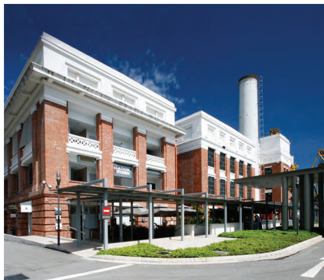
St James Power Station was gazetted as a national monument in 2009.
