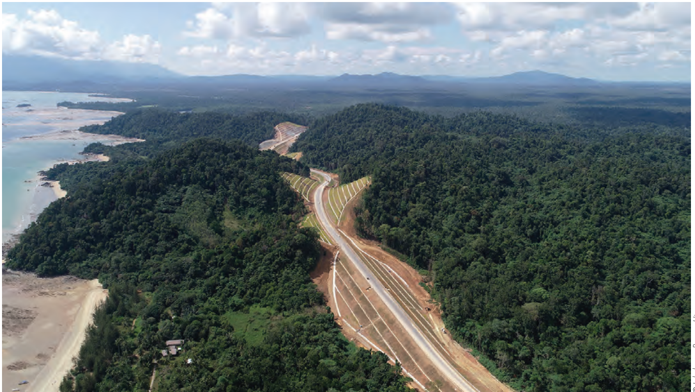
Pan Borneo Highway Sarawak is believed to be the first road and highway project in Malaysia to utilise BIM technology.
