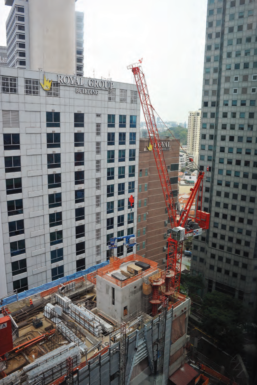
ABOVE AND LEFT: The Potain MCR 295 working on the CapitaSpring. The crane was chosen to help the contractor overcome the project's challenges, such as tight timetable, tall building height and limited space in a congested downtown location.
