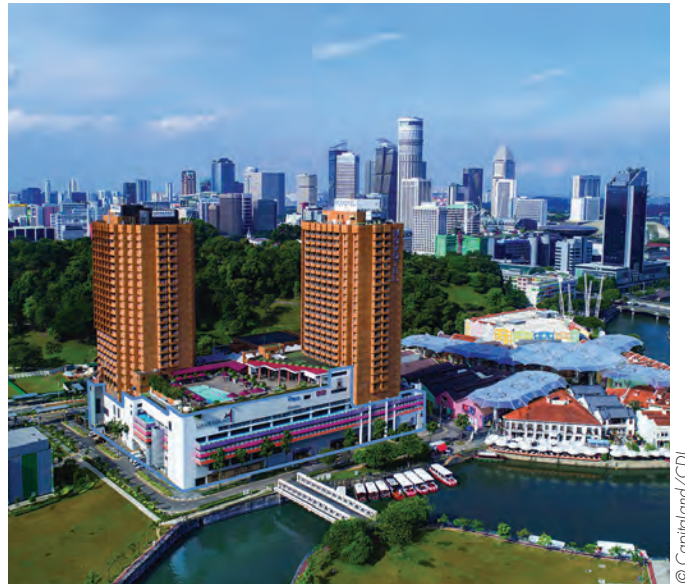
CDL, CapitaLand and Ascott Reit have teamed up to redevelop the Liang Court site in Singapore into an integrated development, featuring 700 residential apartments, a commercial component, a hotel and a serviced residence.
