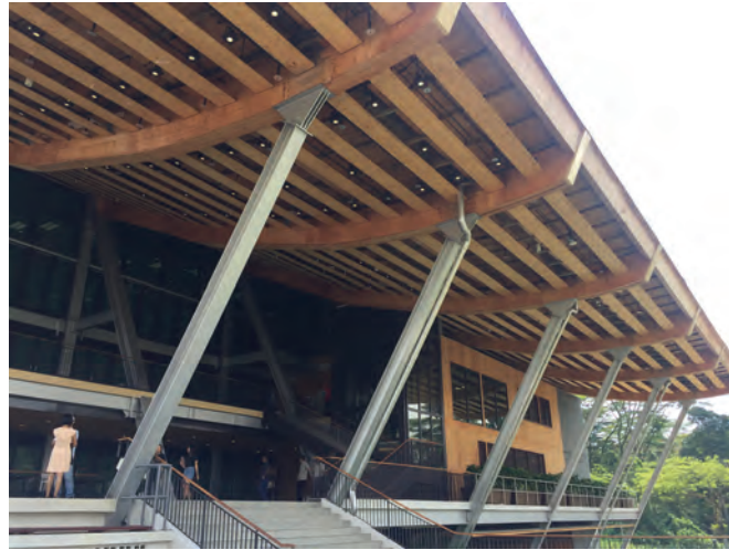
LEFT AND BELOW: The Wave is the sports hall at Singapore's Nanyang Technological University constructed using MET, which was opened in 2017. Now, the university is developing another MET project - Academic Building South - set to be Asia's largest timber building upon completion.
