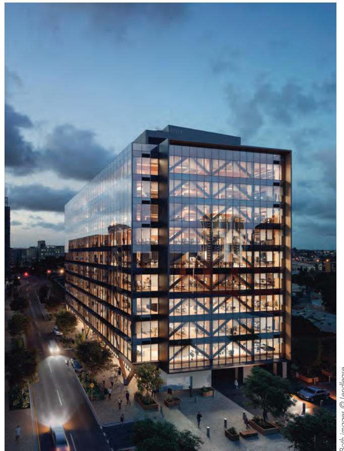
MAIN AND ABOVE: Aurecon has worked on a number of significant timber building projects in Asia Pacific, including the 25 King Street in Brisbane, Australia.
