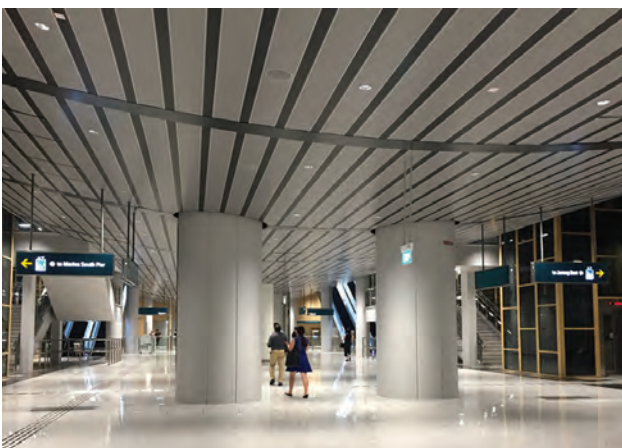
Canberra Station features an extensive use of environment-friendly materials and products. It is the first to be accorded the Green Mark Platinum award under the new Green Mark for Transit Stations scheme recently introduced by BCA.
