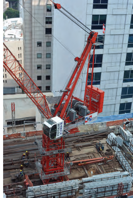
ABOVE AND LEFT: The Potain MCR 295 working on the CapitaSpring. The crane was chosen to help the contractor overcome the project's challenges, such as tight timetable, tall building height and limited space in a congested downtown location.
