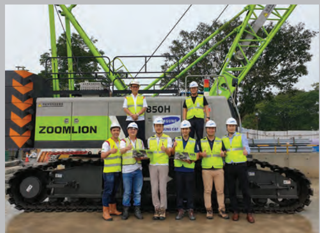
The Zoomlion ZCC850H crawler cranes will be working on the Thomson-East Coast Line MRT project.
